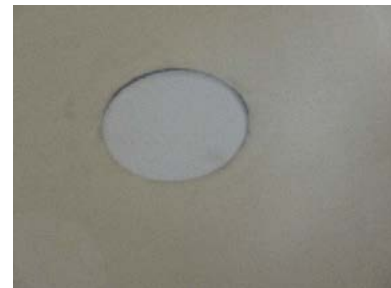
Photo 6.12 Concealed Sprinkler Head
