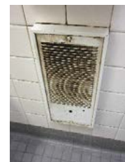
Photo 7.6 Cabinet Unit Heater
