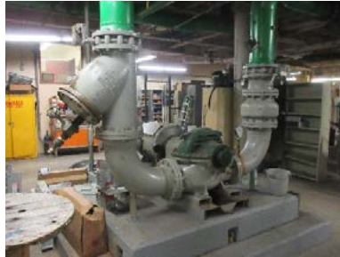
Photo 3.14 – Condenser Water Pump
