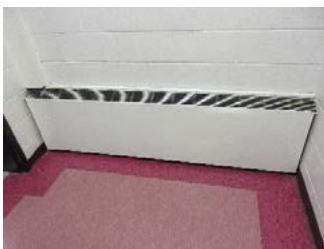
Photo 7.4 Fin tube Radiator
