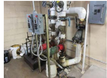
Photo 3.42 – Hot Water Pumps
