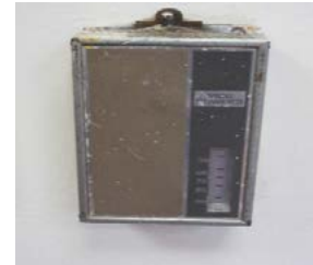
Photo 7.6 Thermostat for Fin Tube in daycare
