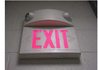
Photo 7.12 Exit Sign / Emergency Wall Pack
