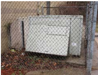
Photo 7.1 Daycare HVAC Unit
