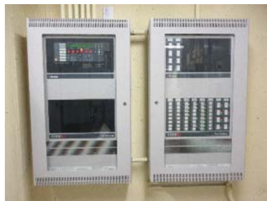
Photo 5.9 Fire Alarm Panel
