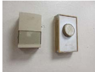
Photo 7.5 – Sensor and Unit Heater Controller
