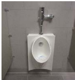
Photo 3.49 Low Flow Urinal
