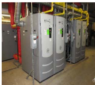
Photo 3.1 - Gas fired boilers
