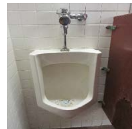
Photo 3.45 – High Flow Urinal
