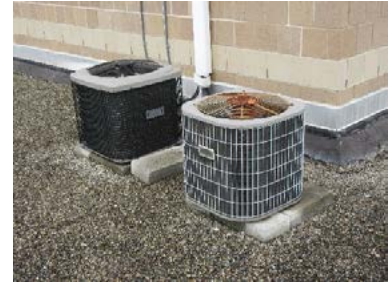
Photo 3.15 – Condensing Unit
