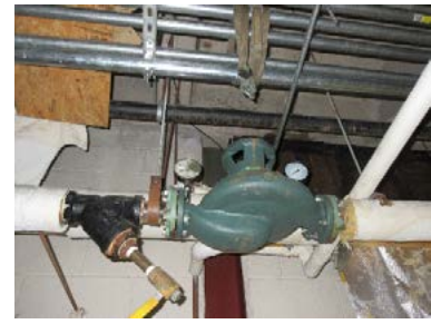
Photo 6.3 – Missing Motor on Pump
