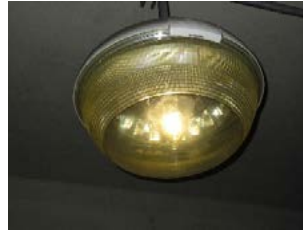
Photo 7.11 – Metal Halide Fixture
