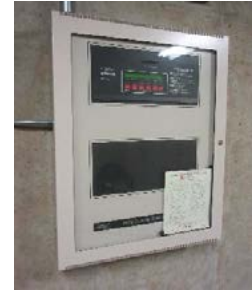
Photo 6.10 Fire Alarm Panel
