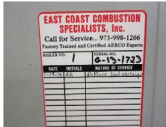
Photo 3.41 – DHW Heater Tag
