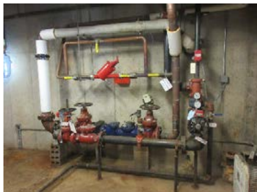
Photo 6.11 Incoming Fire Service
