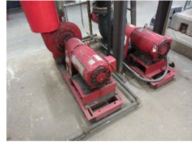
Photo 3.6 – Hot Water Pumps
