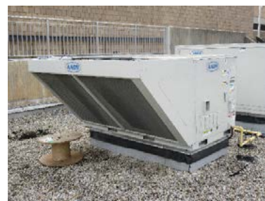
Photo 3.3 – Gas Fired RTU
