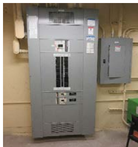
Photo 5.5 - Main Electric Panel
