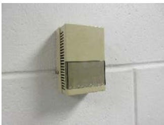
Photo 4.10 Temperature Sensor
