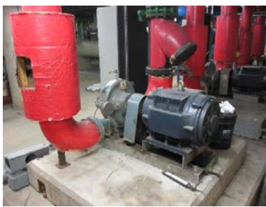
Photo 3.2 – Hot Water Pump
