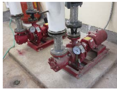
Photo 5.3 – Hot Water Pumps
