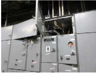
Photo 3.25 – Exposed Wires
