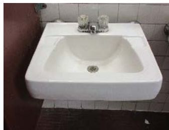
Photo 3.44 – High Flow Sink
