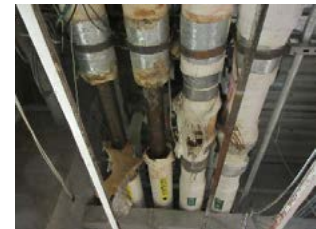
Photo 4.3 Leaky AHU piping
