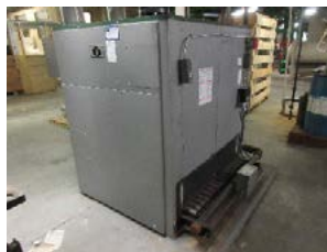
Photo 4.5 – Boiler for Center of Technology
