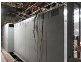
Photo 3.22. – Exposed Wires
