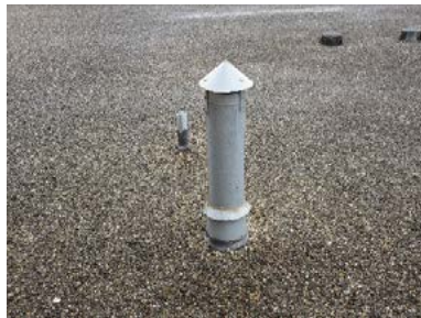
Photo 3.17 – Boiler Vent
