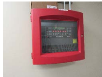
Photo 3.35 – IT Simplex Panel
