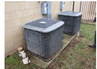
Photo 7.3 Condensing Unit
