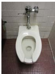
Photo 3.43 High Flow Toilet
