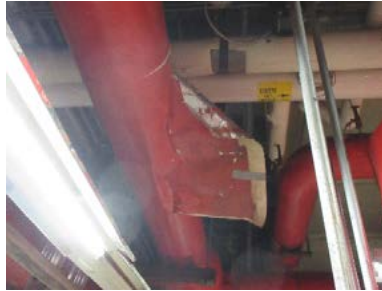
Photo 3.5 – Deteriorating Insulation
