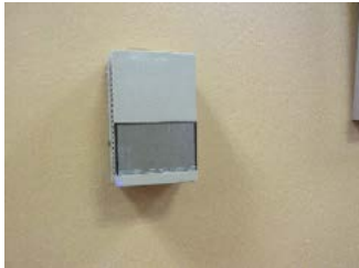
Photo 7.4 Temperature Sensor
