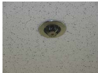
Photo 4.26 Sprinkler Head
