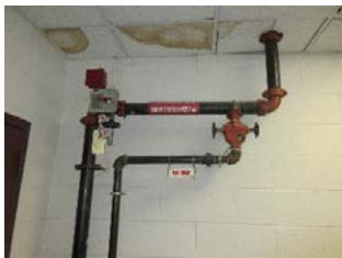
Photo 4.25 Sprinkler Piping
