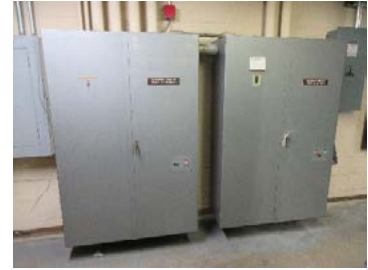
Photo 3.33 – Transfer Switches
