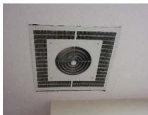
Photo 7.5 – Ceiling Unit Heater
